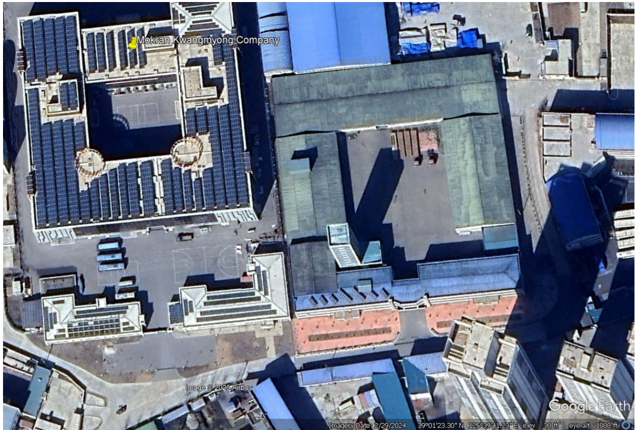
Mokran Building (39° 1'21.33"N, 125°39'34.86"E)
